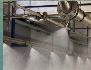
WATER SPRAYING SYSTEM for CAR DECK
