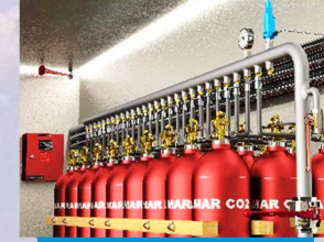
CO 2 FIRE EXTINGUISHER
