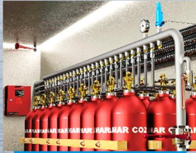
CO 2 FIRE EXTINGUISHER
