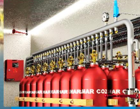
CO 2 FIRE EXTINGUISHER
